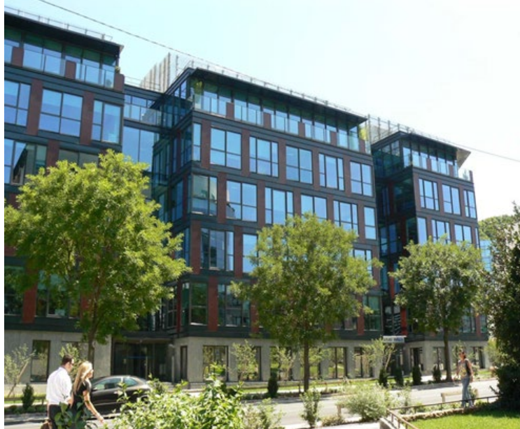
Pic. 6. Facade with Faceactive photovoltaic modules
